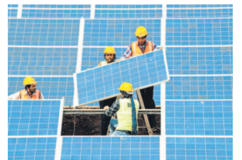
The agreement also includes creation of pumped storage projects of 2 gigawatts.
