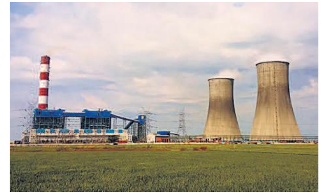
Nabha Power, a coal-fired supercritical power plant, operates two units, each generating 700 MW.
