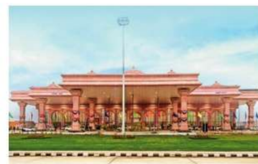
Expanding & upgrading air-connectivity
