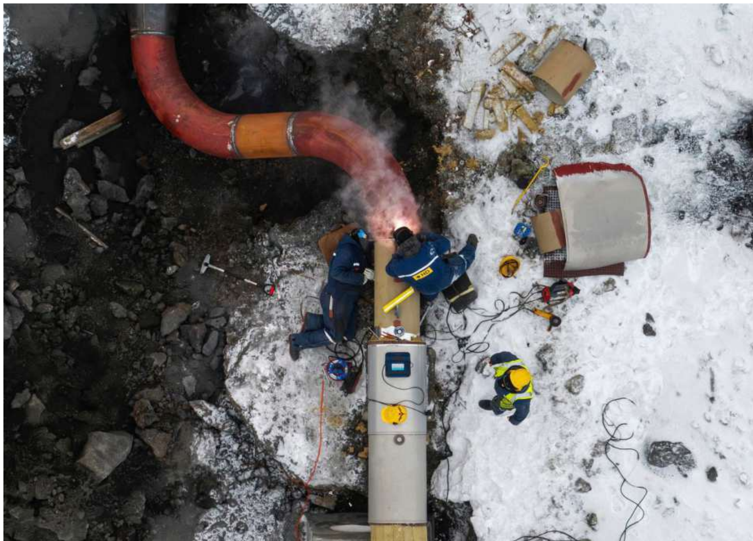
Workers repair a pipeline that carries hot water from the Svartsengi geothermal power plant to the Reykjanes peninsula, in Grindavik, Iceland, February 9, 2024. Repairs on the pipes went on overnight in temperatures as low as minus 14 degrees C, utility company H.S. Orka said, after they were damaged by a volcanic eruption in southwestern Iceland.
