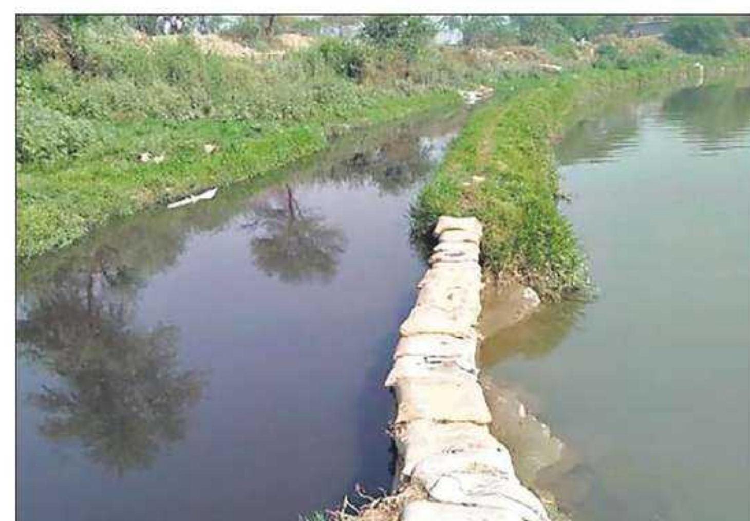
Drain six was found to be overflowing into drain eight. HT
