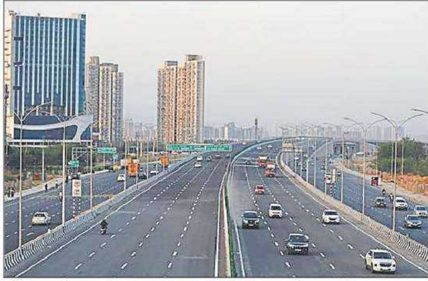
The Gurugram section of the Dwarka expressway was opened for traffic on Tuesday. PARVEEN KUMAR/HT PHOTO
