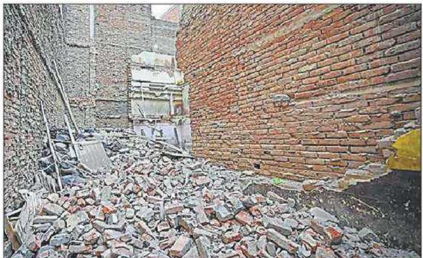
The two-storey building which collapsed at Kabir Nagar in northeast Delhi on Thursday. SANCHIT KHANNA/HT PHOTO
