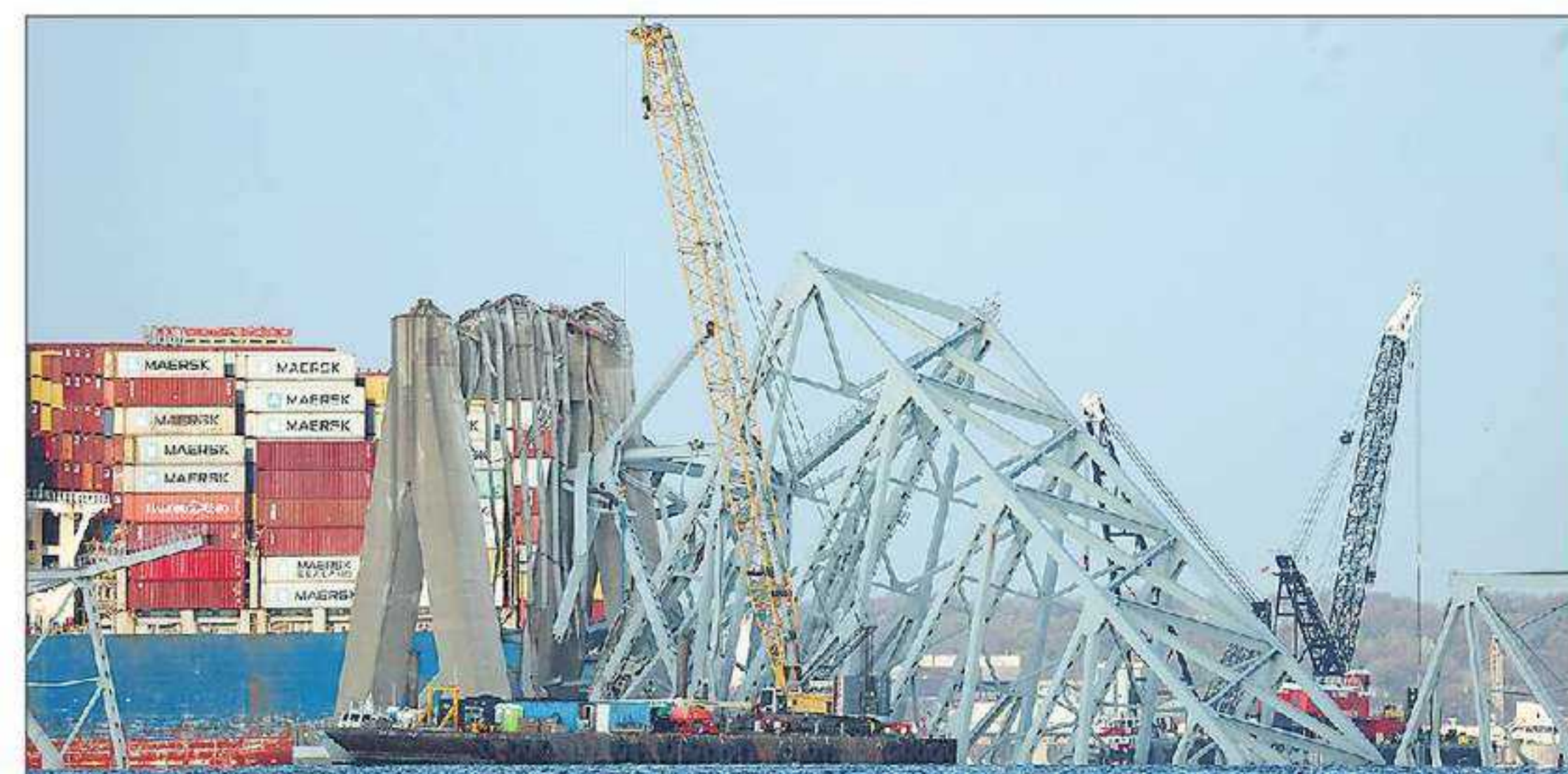
A crane works on the debris of the Francis Scott Key Bridge, which collapsed after a container ship crashed into it, on Friday in Baltimore. AFP
