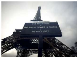
A five-day strike at the Eiffel Tower this month brought attention to the monument's bad state of repair. REUTERS
