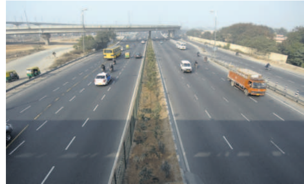
Since 2018, NHAI has successfully completed six rounds of the road asset (bundle of roads) monetization through ToT mode. MINT
