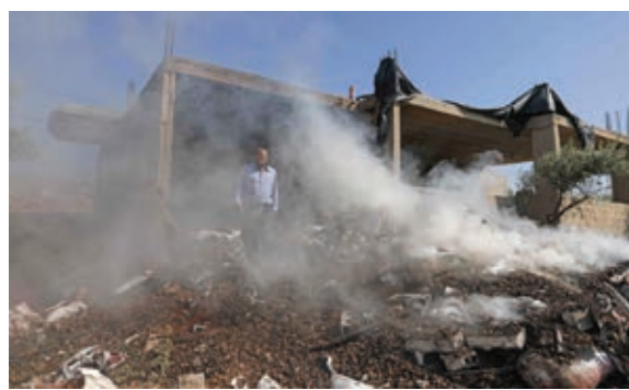
A Palestinian inspects the damage to a home in the village of Mughayir near Ramallah in the Israeli-occupied West Bank, on Saturday. — AFP
