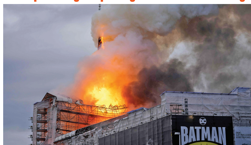
A fire rages through one of Copenhagen's oldest buildings on Tuesday, causing the collapse of the iconic spire of the 17th-century-old stock exchange. The building, one of the oldest in the Danish capital, was undergoing renovation work when it caught fire, whose cause was yet unknown. ■ Report on Page 6 — AFP
