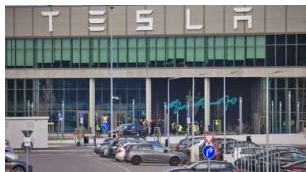
IMPACT. Tesla had 140,473 employees globally as of December 2023, the reported cuts will affect about 15,000 workers
