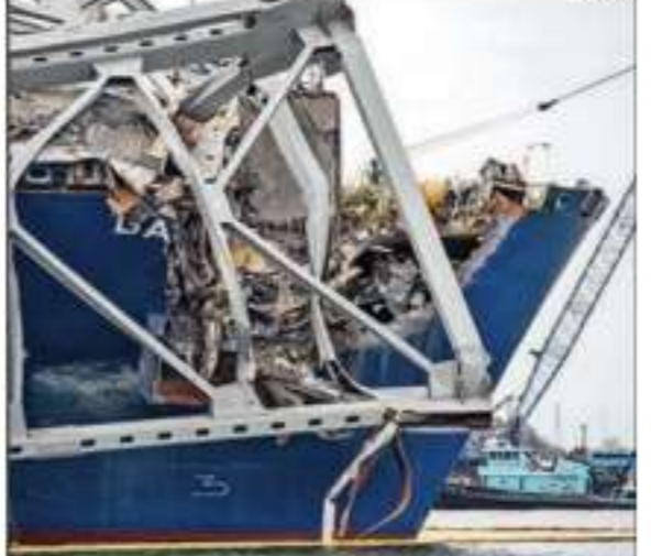
A portion of the collapsed Francis Scott Key Bridge
