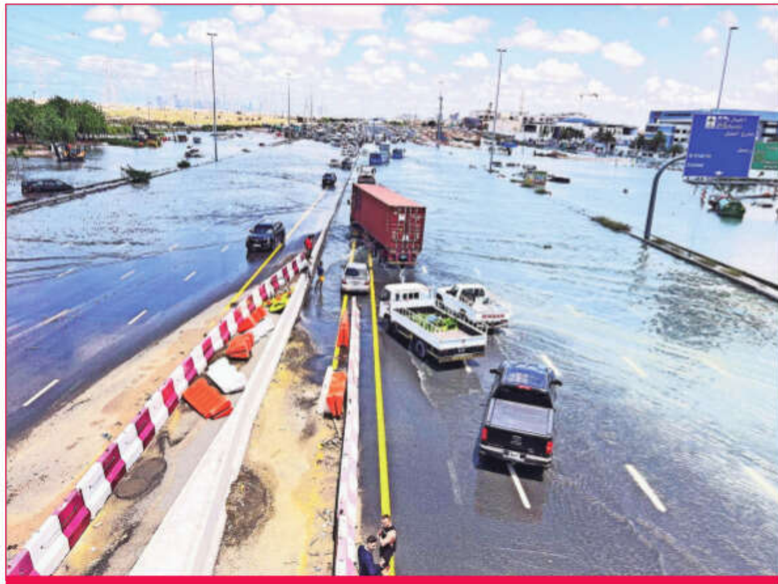
Cars are stuck on a flooded road after a rainstorm hit Dubai on Wednesday. Authorities and communities across the UAE were clearing debris after at least one person died and homes and businesses were damaged in a rare torrential storm
