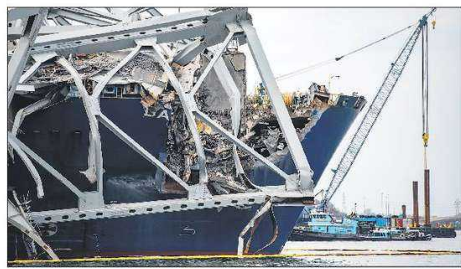
A section of the collapsed bridge on the container ship Dali. AFP
