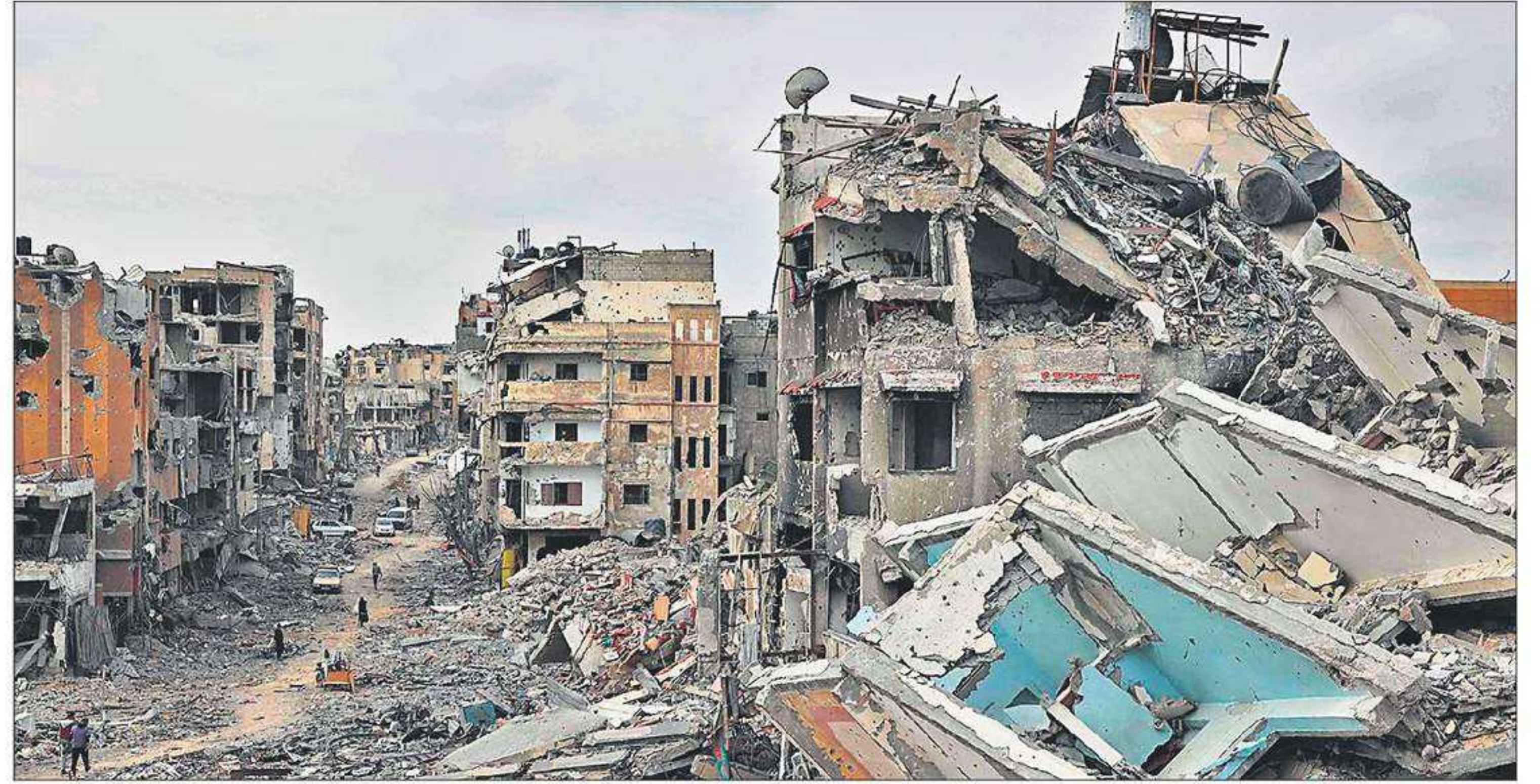
Palstinians walk past damaged buildings in Khan Yunis on April 8, after Israel pulled its ground forces out of the southern Gaza Strip, six months into the devastating war sparked by the October 7 attacks.
