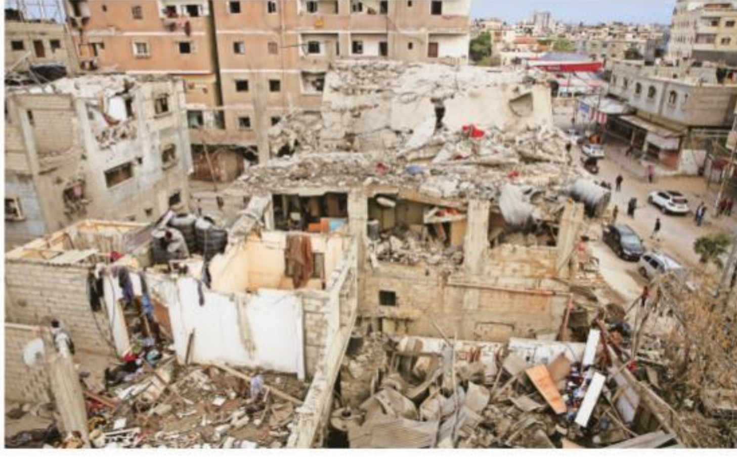
Houses destroyed in Israeli strikes in Rafah in southern Gaza on Monday. Reuters
