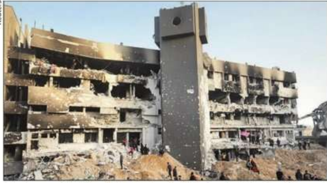
The damaged building of al Shifa hospital after Israel military's withdrawal
