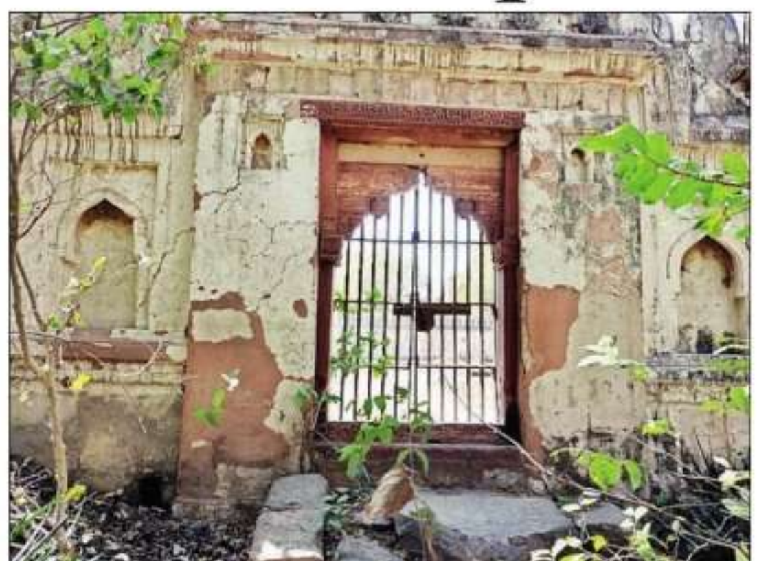
The 16th-century Jamali-Kamali tomb (left) and mosque (centre) in the Mehrauli archaeological village complex; the wall that remains of the Balban's tomb complex (right) will also be conserved
